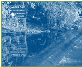
Warning sign at Broadmeadows lowhead dam. Photo courtesy of Ellie Nowels
